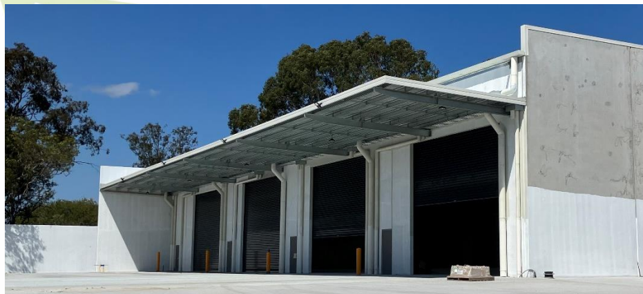
The painting of the building has begun
