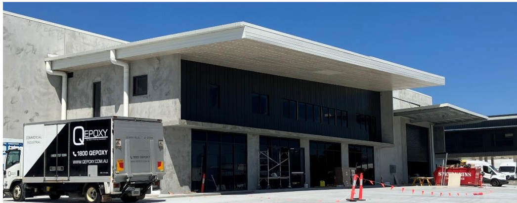
The soffit is fully installed
